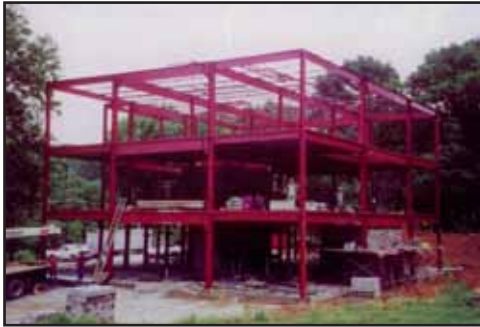
Nashville corporate building under construction
